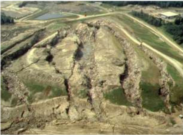
(a) Multiple rotational failure (500,000 m<sup>3</sup>)
