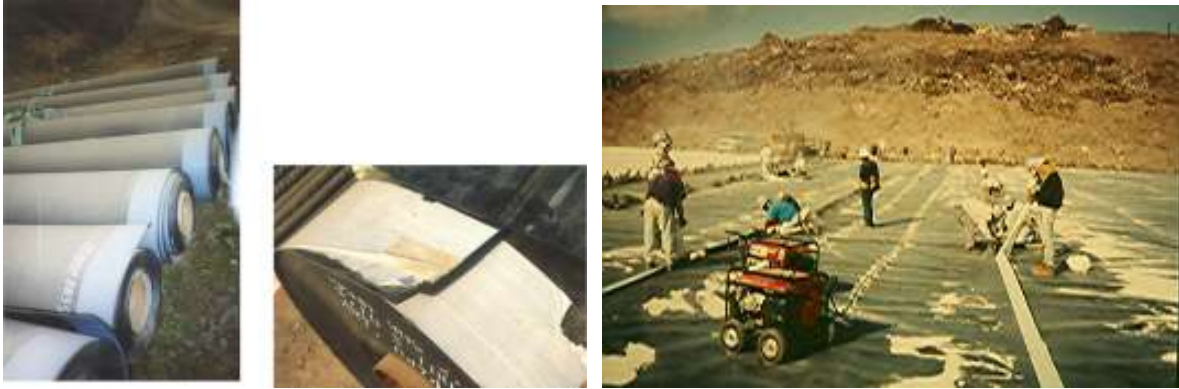
(c) Geomembranes with taped edges
