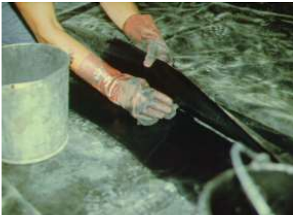
(a) Cleaning area for seaming
