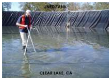
(b) Water covering geomembrane
