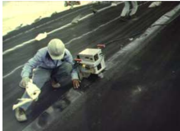
(b) Drying an area for seaming
