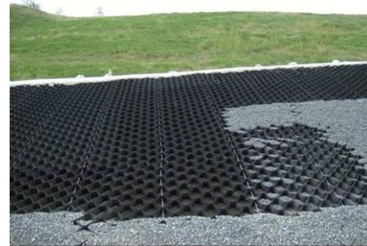
Diagrams and photographs of three-dimensional geocells used for civil engineering applications. (Compliments of In-Line Plastics/GeoProducts, Syntec Corp. and InterGeo/Golder)
