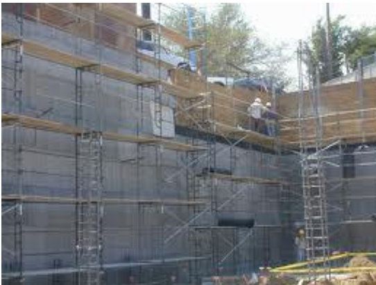
(c) Temporary retaining walls (comp. J-Drain)
