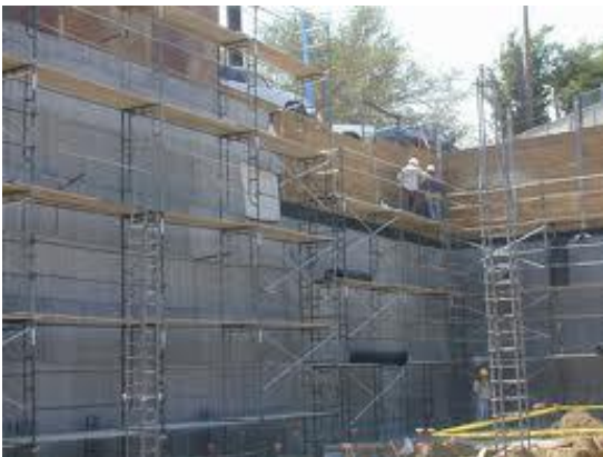
(c) Temporary retaining walls (comp. J-Drain)
