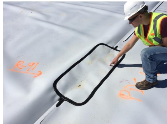
Fig. 2 Extrusion fillet welded patch over sampled area. (GSI Photo)
