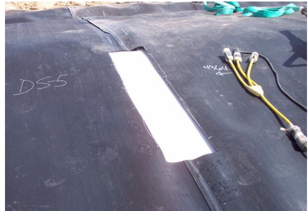
Fig. 1. Area of seam sample removal. (GSI Photo)
