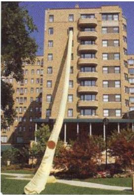
The advanced modular evacuation system is triggered by a fire alarm; the chute unfolds automatically from the structure. The user enters the chute through automatic doors and slides down, landing on a cushioned landing pad. Acceleration during descent is controlled through a series of “steps,” which occur every five floors.
