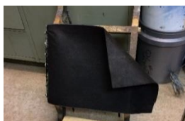
Bad clamping of a geocomposite
