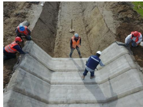
Installation of GCCM as a canal lining
