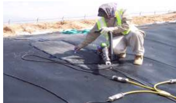
(b) Repair patch placed over previously cutout destructive seam location
