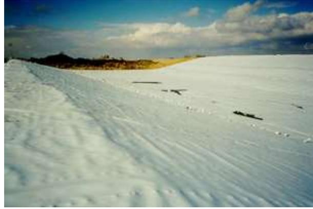
(b) Co-extrusion white surfaced sheet
