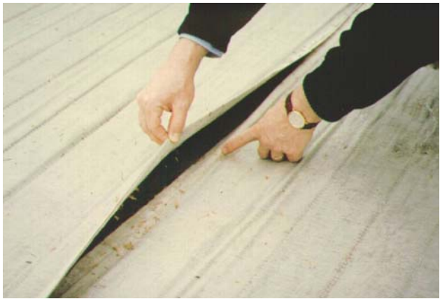
(a) Loss of initial overlap - no separation, hence, not included in Table 1
